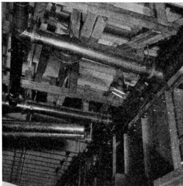
Fig. 9—Quarter and half-wavelength line sections used to form high-"Q" filter elements preventing cross coupling of "sound" and "picture" transmitters separated a few percent in frequency and operated on a common antenna.
