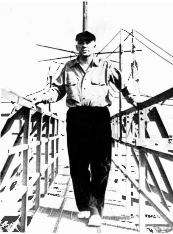
*The inventor is shown on the catwalk of his 400-foot experimental FM antenna, built in 1938 on the Palisades high above the Hudson River at Alpine, N.J. He opened station W2XMN at this site in 1939, the first high-powered FM station, the only previous one having been a low-powered amateur station used for demonstration purposes.*
