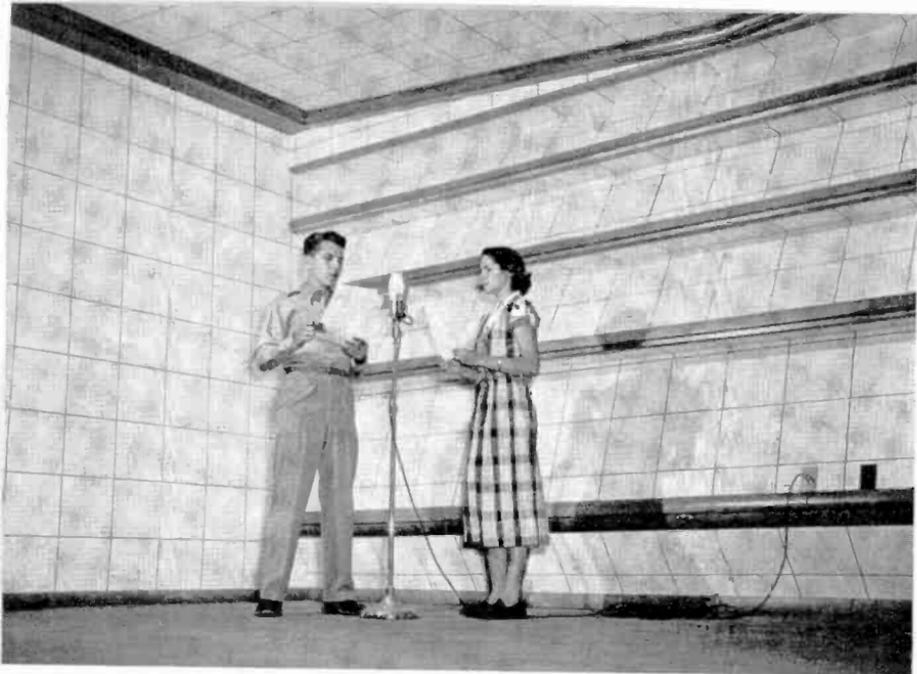
11. Saw-Tooth Wall Construction for Extreme Acoustic Deadening.
