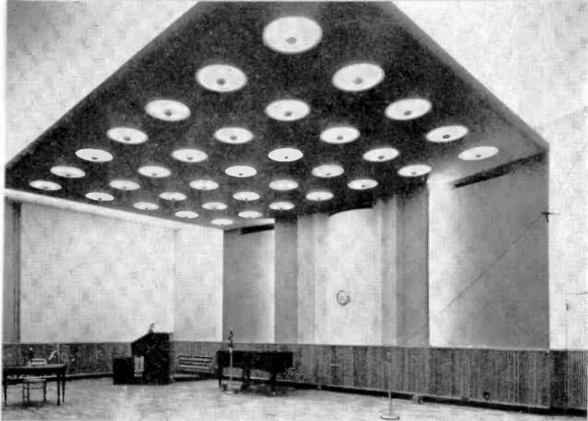
9. Dual AM-TV Studio, 33'  $\times$  45', Two Stories High. It can be adapted for either radio or TV productions; walls include "splayed wing, as well as cylindrical reflectors. Resilient, squeakless floor is made by 1' lengths of tongue-and-groove beech, fitted and held in place by mastic. An acoustical canopy is suspended above the work area. (Photo by courtesy of WGN, Chicago.)
