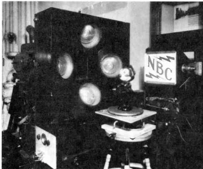
*During the early experiments with electronic television, RCA laboratories used, as a moving object to televiser, a 12-inch paper maché model of a popular cartoon character, Felix the Cat, posed on a revolving turntable under hot lights. The image at left shows how Felix looked on television in 1929 when picture definition was still only 60 lines per frame.*
