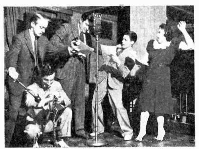
Fig. 21.—Dramatic east and sound men. Notice the use of the eight-ball mike to pick up the sound of the chains, while the revolver is held to one side of a ribbon mike. Also notice the physical acting of those who are participating in the play. The girl screaming is at the dead side of the microphone.
