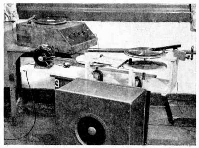
Fig. 48.—Student-constructed variable-speed turntable.
