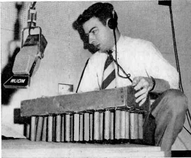
FIG. 48. The sound of men marching is being made with equipment constructed for that purpose. It is generally advisable to have a suspended mike for sound, no part of which rests upon the surface from which the sound is being generated. Notice the box is used with an end-to-end motion, not vertically up and down.
