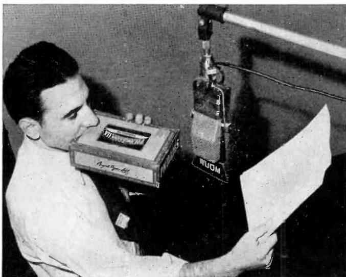
FIG. 50. Actor using a muffle box, which is a cigar box with a half-moon cut out of the end, to create the effect of a person speaking from behind a closed door or of an off-stage voice.
