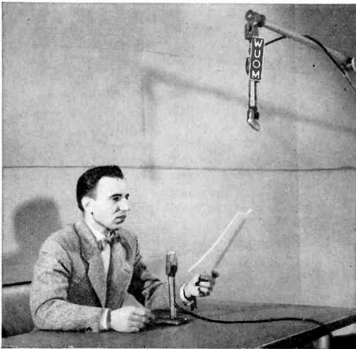
FIG. 29. Announcer's setup. Program being broadcast over AM station through Bantam microphone on table and fed to FM station through microphone on boom. (*University of Michigan.*)
