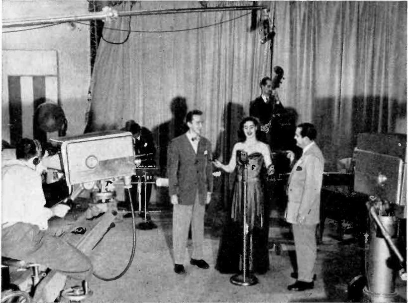
FIG. 34. The television soloist in this picture is being picked up for television by the microphone above her head. The ribbon mike on the standard is a part of the stage setting. (*General Electric.*)
