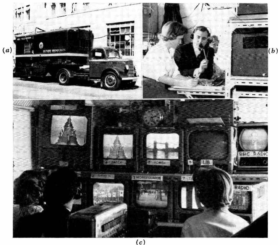
Fig. 20-35. Main BBC control center for the royal wedding. (a) Outside Broadcasts van outside Broadcasting House. (b) Peter Dimmock, head of Outside Broadcasts, at control desk with two assistants. (c) Mr. Dimmock faces an array of 10 monitors displaying the various inputs and outputs to the switching center. Pickup from the Tower Bridge (top center monitor) does not show on the chart. The purpose of this was to show the royal yacht leaving for the honeymoon.
