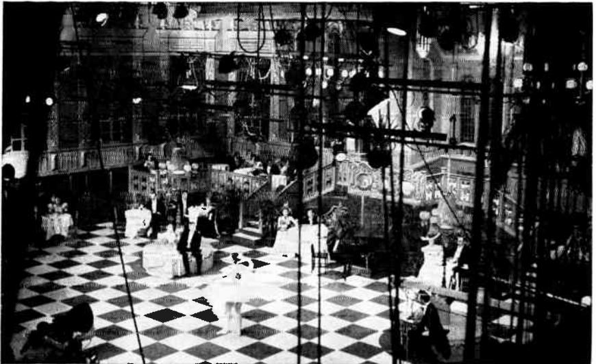
Fig. 18-11. Lights mounted on counterweighted battens (ABC-TV, New York, Studio 1).
