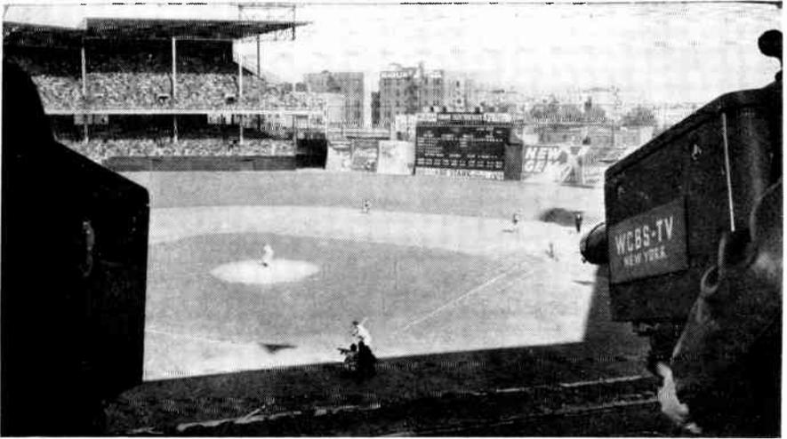
Fig. 20-33. Two CBS cameras cover the play at Ebbets Field from behind home plate. An early photo, this picture shows the cameras in use without electronic view finders.
