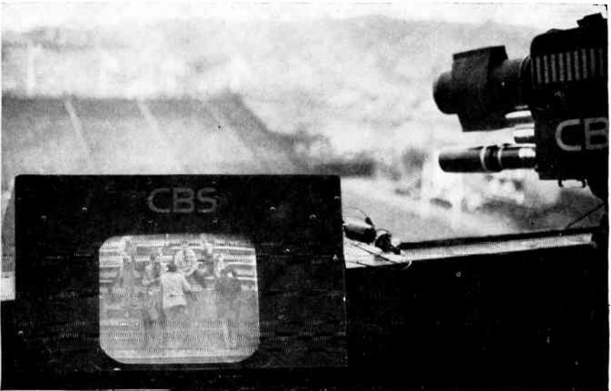
Fig. 5-5. Video Reflector lens (early model) focused on people in the stands across a football field. The camera's picture is visible on the monitor in the foreground.
