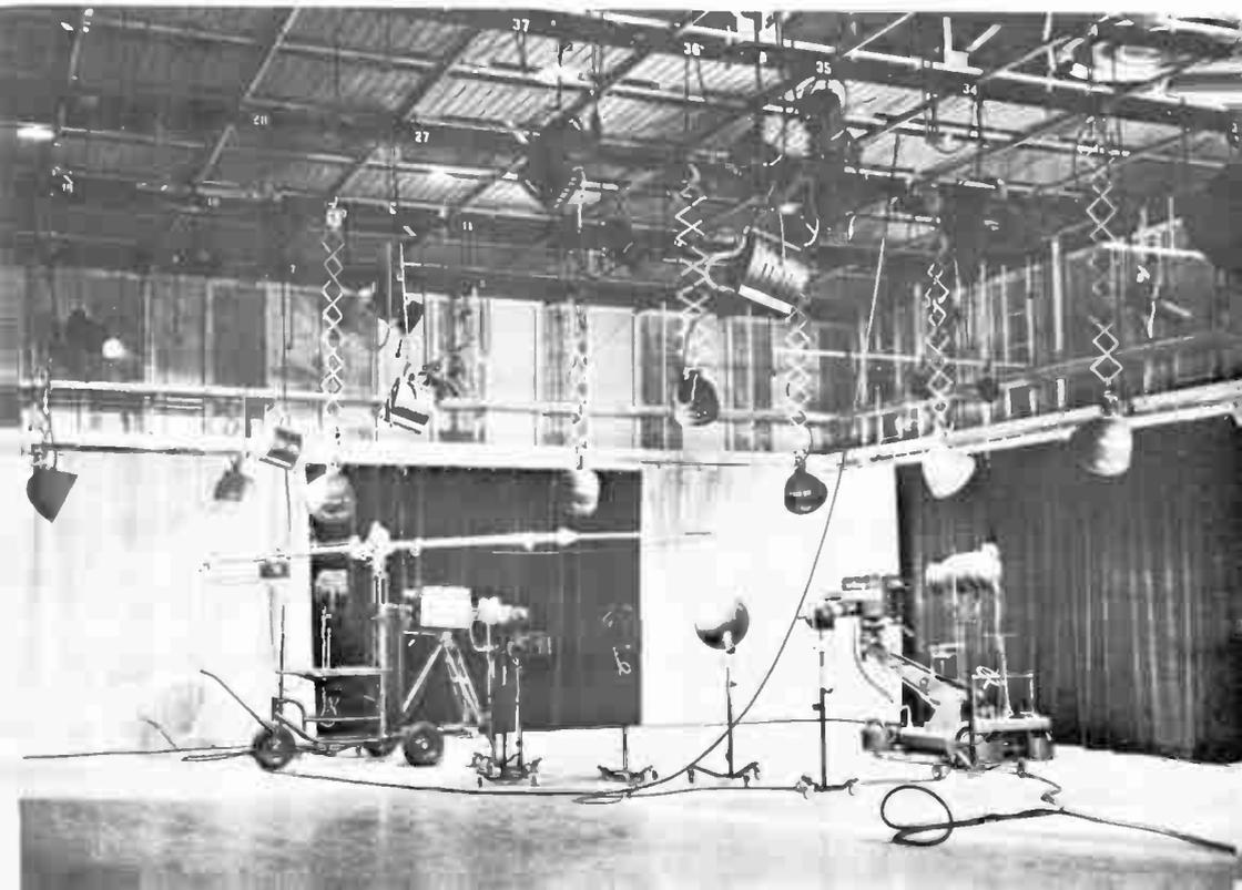
performers or objects, may be floor banks or single-unit scoops or fresnels. Fixed or focusing spots are used for *highlighting*; that is, bringing some object in the picture into special prominence. Crossed spots can highlight a merchandising display and at the same time counteract each other's shadows.
