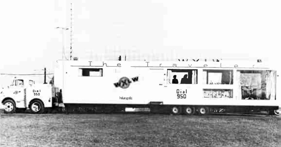
Figure 4. Radio Mobile Unit, WXLW, Indianapolis (Indiana). Completely self-contained with studio, relay unit, and living facilities.
