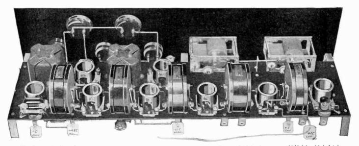
The photograph above shows an eight-tube super-heterodyne set of extra fine quality. Each of the heteroformers are shielded in nickel-plated metal shields. The two variable condensers for tuning the aerial and oscillator circuits should he of the straight line frequency type. The two audio frequency transformers are extra large concert type, the first stage of audio being all that is necessary for average reception on a loud speaker.
