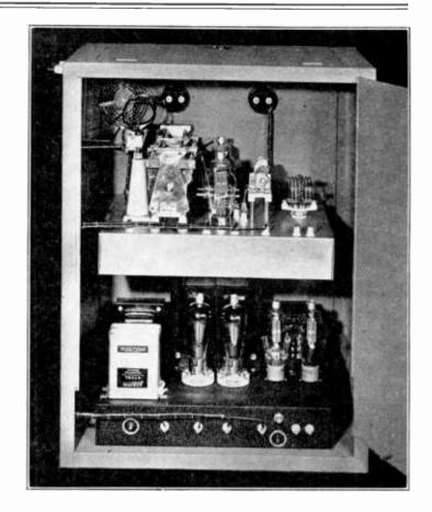
ments.  $S_4$  controls the plate voltage to the final amplifier and modulator.  $S_3$  is a safety "door switch" in series with the primary of the plate transformer. This switch is located on the rear drop of the chassis and closes only when the rear door of the rack is closed. It is operated by the long machine screw visible on the inside of the rear door in Figure 14.
