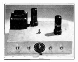
Figure 12. DUAL FREQUENCY CRYSTAL CALIBRATOR.
