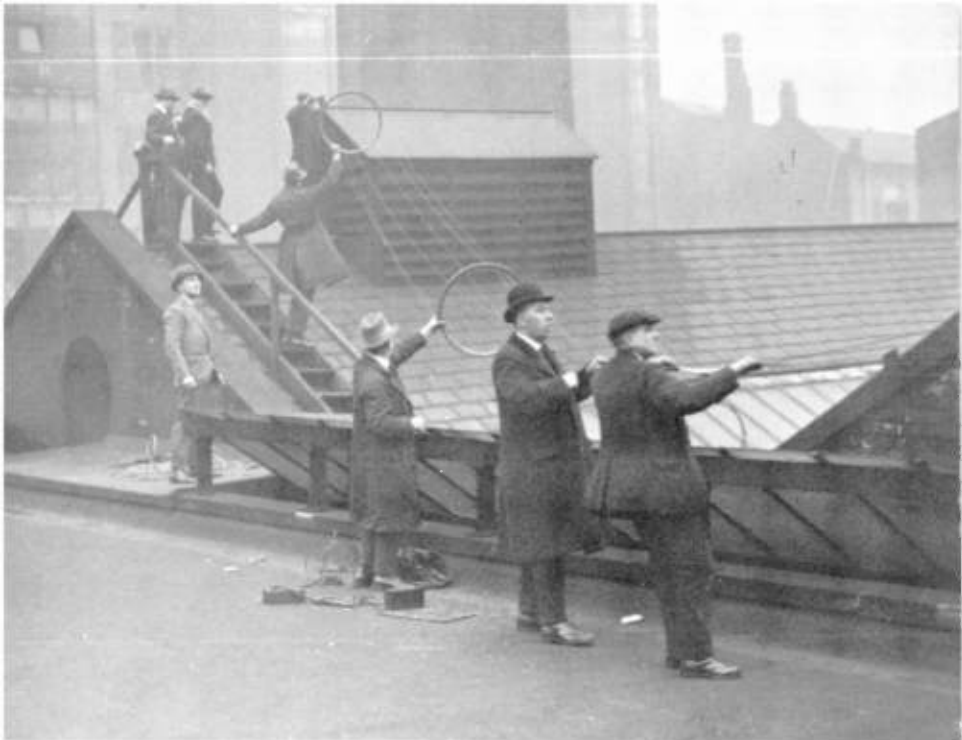
4. Robert Wood (left, in light suit) supervises the installation of the 'sausage-hoop' aerial on the roof of 2ZY, the BBC's Manchester station, on 28 January 1924.
