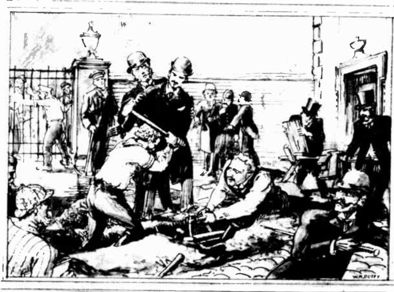
*Figure 7.5 Ferranti chisel test—on a live 10 kV cable*
