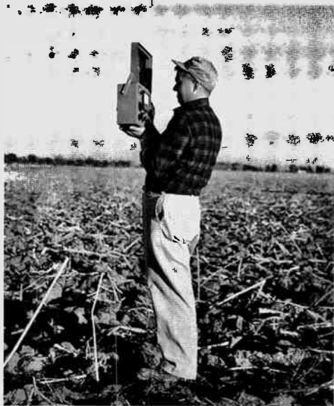
Ralph Evans, Sr., taking field strength readings. (Courtesy of Ralph Evans, III)
