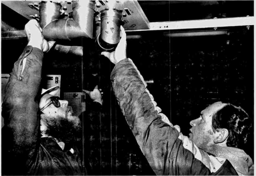
Nolan Tobias (left) and Don Kay install the cooling line for the old WMVT transmitter. Tobias donated all of the time needed to install the unit. (VCY America photo)
