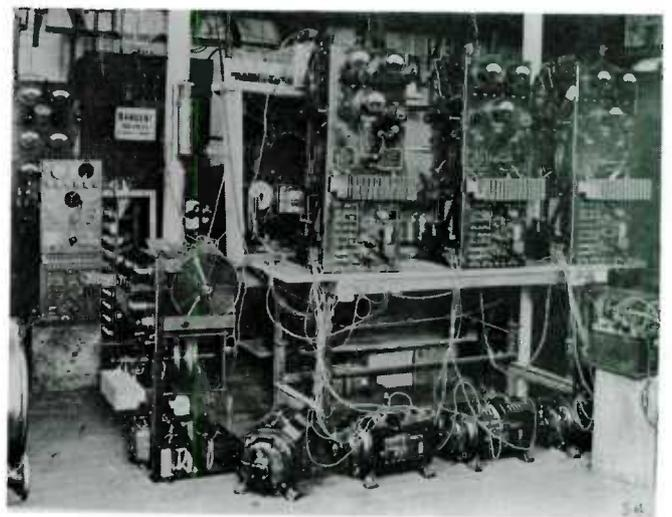
Testing quenched-gap transmitters, about 1919.
