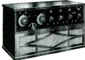
This cabinet is equipped with the model X panel, the same four-tube outfit, mounted in a special cabinet with amplifying horn incorporated therein, and can be used with head phones or single loud speaking receiver, such as the Baldwin type "C." Price of this four tube outfit is.....\$70.00.
