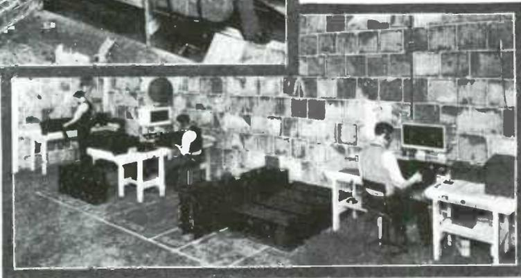
At the left is shown a testing room for completed receivers. Each set, after it is assembled, must be tested over the broadcast range wave-lengths; actual local and distant reception is obtained to assure that it has suitable sensitivity and volume for distance getting.
