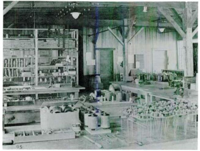
Assembly of SCR74 "trench" transmitters, 1918
