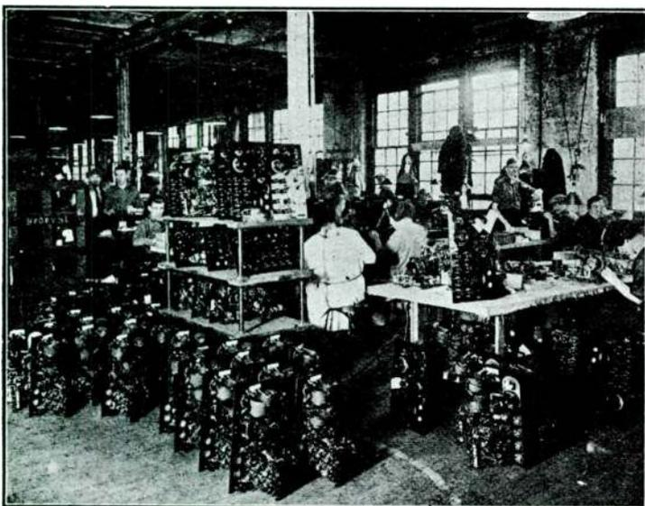
A corner of the assembling room where Federal 61's are made.
