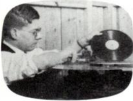
Baird's Phonovision: a recording is about to begin as J. D. Percy puts a wax record on the turntable/scanner.
