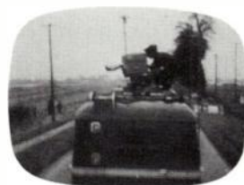
Television coverage of horse racing was transformed by the use of cameras attached to the roofs of vans which drove along the side of the course at the same speed as the horses; hitherto, viewers had been able to see only the winners flashing past the finishing post.
