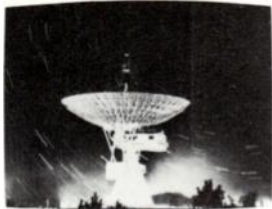
A huge parabolic antenna 50 miles north-east of Tokyo, 30 metres in diameter, used for relaying television pictures of the Tokyo Olympics in 1964 to North America and Europe via the Syncom 3 communications satellite.
