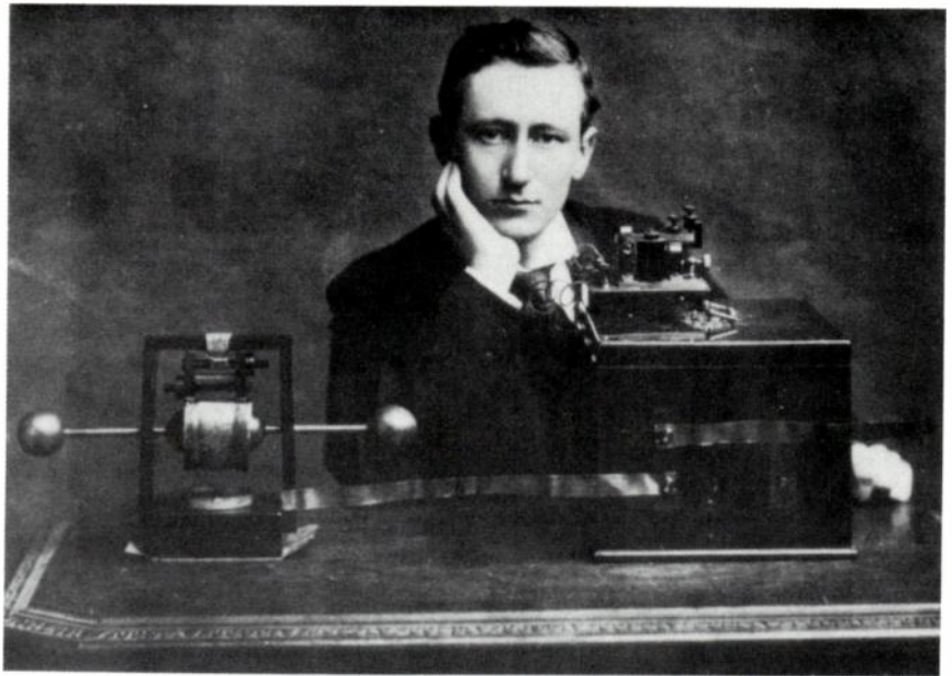
Guglielmo Marconi in England with the mysterious black box which he brought from Italy in 1896. His wireless system consisted of a spark gap transmitter and a coherer receiver.
