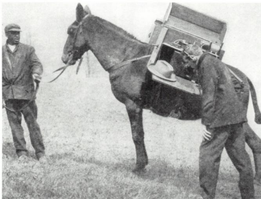
Early experiments with the De Forest portable wireless telephone at Newark, New Jersey.
