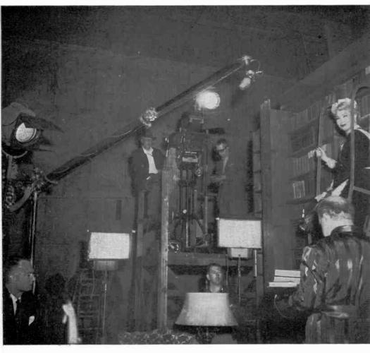
FIGURE 5. TV FILM TAKE. To take a high-angle shot, the camera has been placed on a platform. Lighting shown consists of two fill-lamps, center, and fresnel lamps, left and top, with "barn door" shutters. The boom mike can be moved from side to side, extended or retracted, and raised or lowered. (Photo courtesy of CBS Television)
