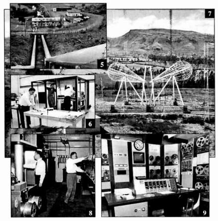
5. The powerhouse and dual penstocks after completion of the second hydroelectric plant in 1982, which boosted the electrical power output to six million watts.
