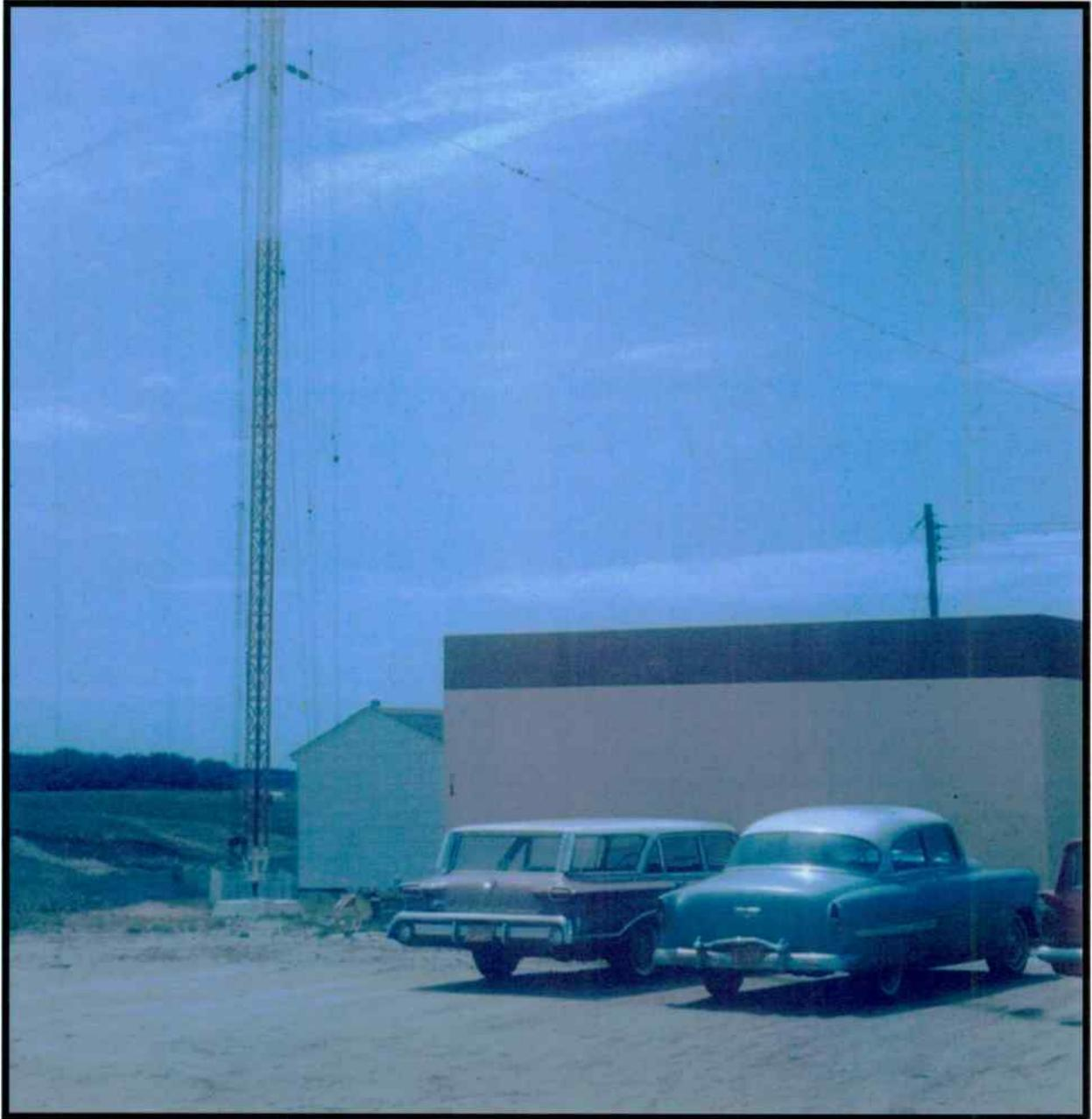
***Another shot of the FM tower installation. In this picture, one can see better the misalignment still present in the uprightness of the tower. The vehicles in front belonging to KWNS employees. Still unknown at this time was the effect the new grounded FM tower was going to have on the AM patterns.***
