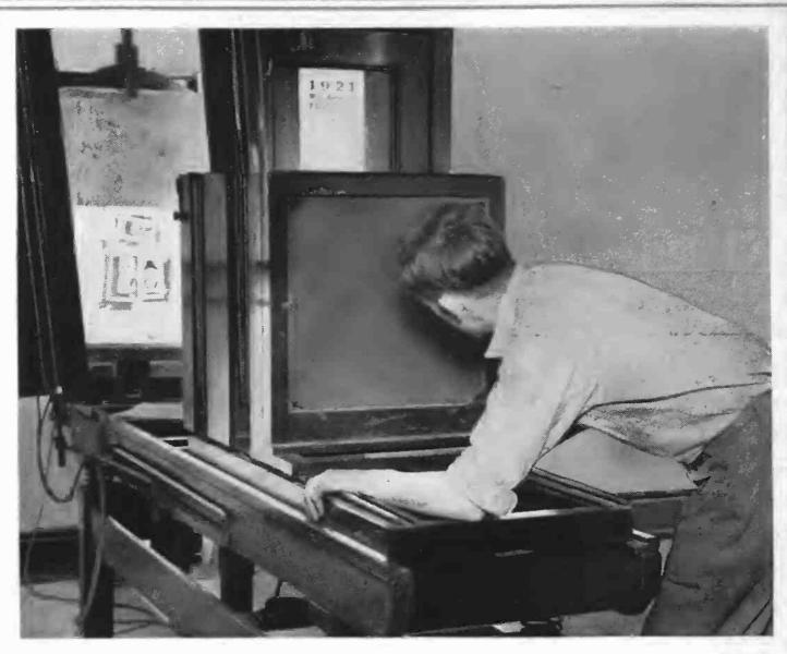
The first step in making an engraving is shown above—photographing the original. Below, the etcher has just taken the zinc plate out of the acid bath after a "bite."
