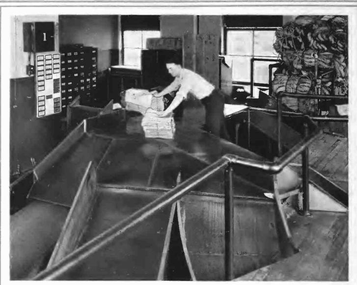
A BELT conveyor throws bundles of papers up on this platform. The workman notes the tag on each and pushes it down the proper chute into waiting wagon or truck.
