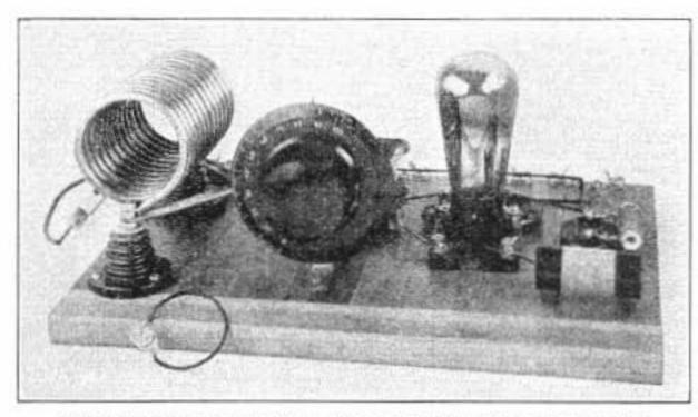
THE SINGLE-CONTROL LOW-POWER TRANSMITTER The plate tank circuit is at the left. The grid coil, leak and grid condenser are to the right of the Type '10 tube.
