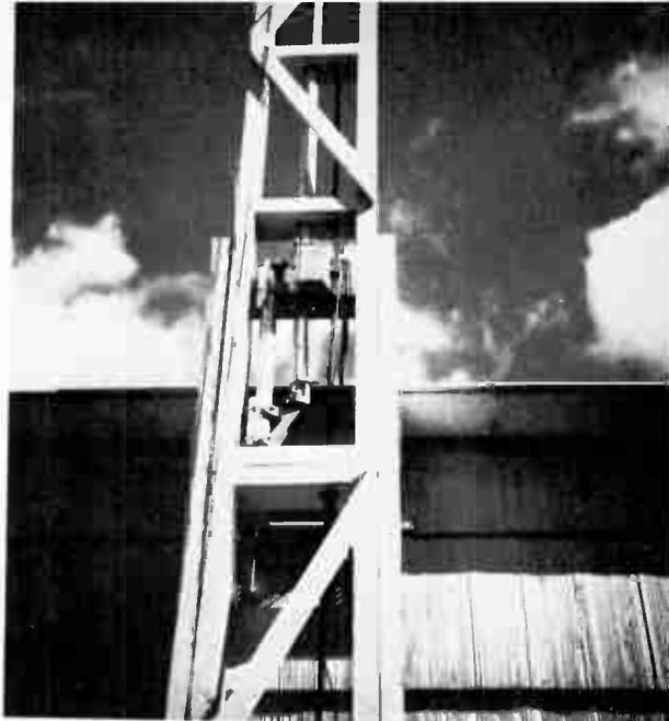
Fig. 21-67 — This close-up shows the rotator and cable installations. A double 2 X 4 is used as the base support for the rotator.
