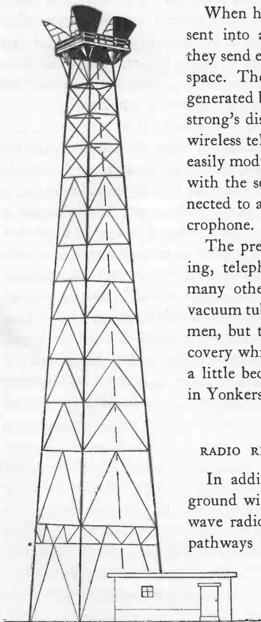
When high-frequency oscillations are sent into an antenna or aerial system, they send electromagnetic waves out into space. The high-frequency oscillations generated by an audion tube using Armstrong's discovery proved to be ideal for wireless telephony because they could be easily modulated or varied in accordance with the sounds of the voice when connected to a telephone transmitter or microphone.
