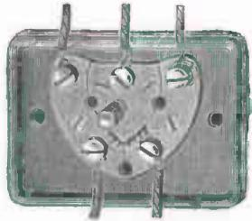
FIG. 99. — Lightning-Arrester and Ground-Wire Switch.
