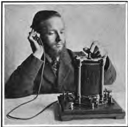
FIG. 97.—Bellini-Tosi radio-goniometer for directive wireless telegraphy.
