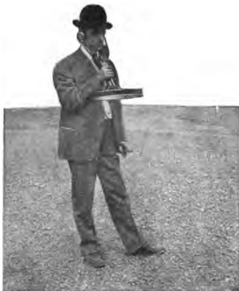
FIG. 141.—Wireless telephone receiving apparatus (induction method).
