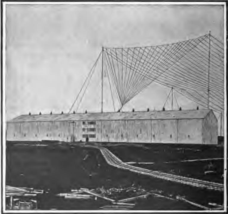
FIG. 153.—The aerial system of a transatlantic station.
