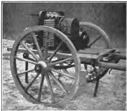
FIG. 101.—Telefunken wireless cart, showing transmitter.
