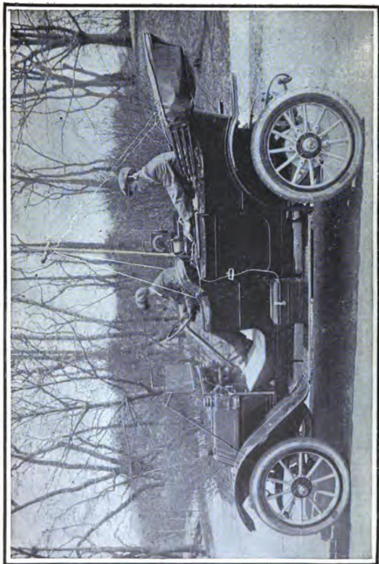
FIG. 106.—Wireless equipped automobile.
