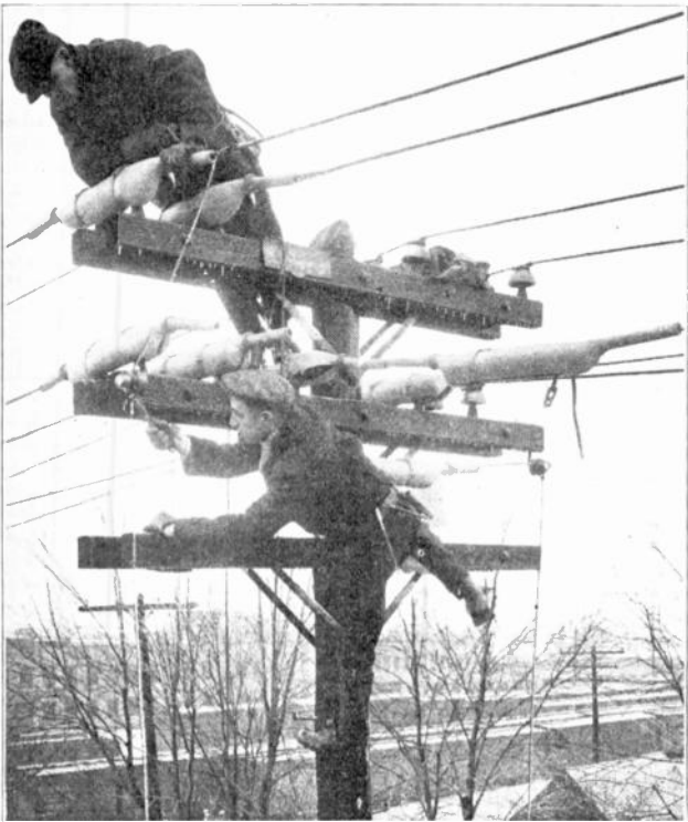
Fig. 368. This photograph shows the use of rubber line hose or "pigs" to protect linemen when working on live transmission or distribution lines. Photo Courtesy Lineman Protector Company.
