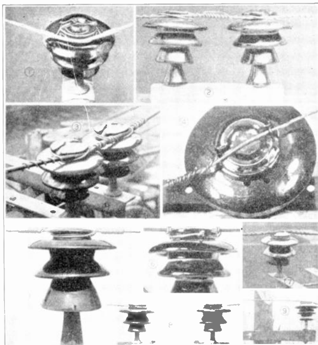
Fig. 334. Above are shown a number of common types of line ties used for attaching conductors of transmission and distribution lines to pin type insulators. Examine each type very carefully as you read the accompanying descriptions and also compare them with the sketches in Fig. 335. Courtesy Lapp Insulator Company, Inc.
