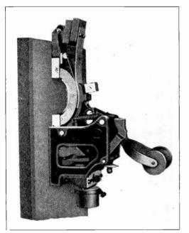
Fig. 66-A. This photo shows a common type of air circuit breaker in closed position. Note the manner in which the main contacts and auxiliary contacts connect with the stationary contacts on the panel.
