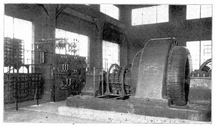
Fig. 156. This photo shows a 3000-h.p., 375 RPM, A. C. induction motor in use in a steel mill. Note the control panel and resistors for starting and speed regulation shown in the left of this view. (Photo Cour.esy General Electric Co.)
