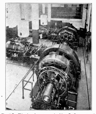
Fig. 41-B. This view shows two engine-driven D. C. generators in a power plant. Two or more machines of this type are commonly operated in parallel.
