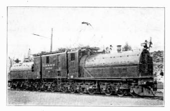
Fig. 3. Electrical locomotives of the above type often use six or eight powerful D. C. motors to turn their driving wheels.
