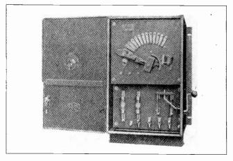
Fig. 124. Speed regulating controller with fuses and line switch enclosed in a controller box.
