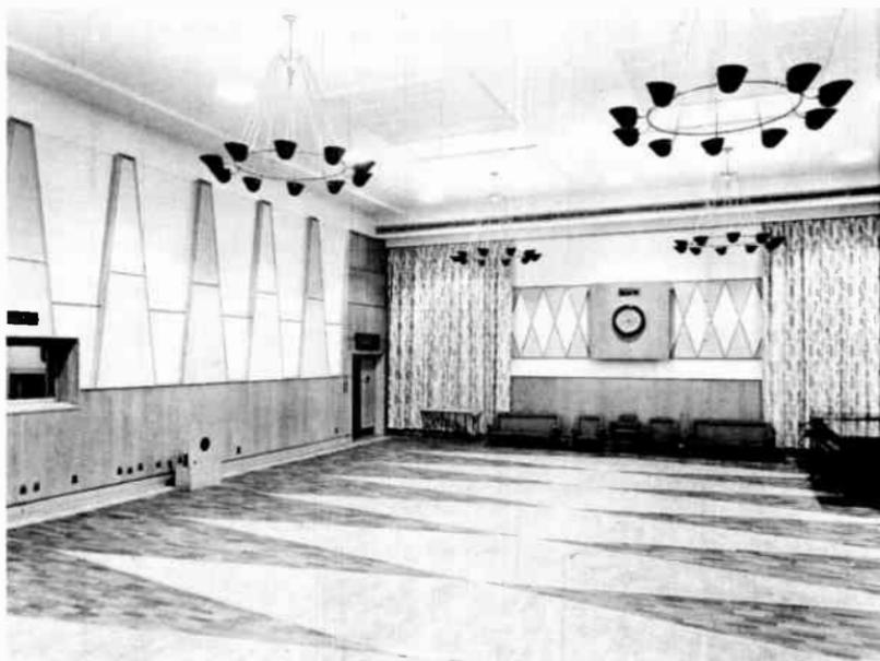
FIG. C/15. *Maida Vale Studio 3, showing acoustic curtains in background and absorbent panels of special shape on side walls and ceiling. The wooden panelling near the floor provides low frequency absorption. Note baffle mounted talk-back speaker on the left.*
