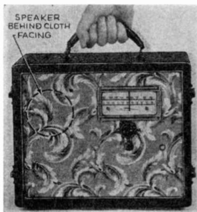
Panel of 4-tube broadcast band portable.
