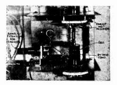
A close-up of an R.F. stage, showing an easy method of ganging condensers.
