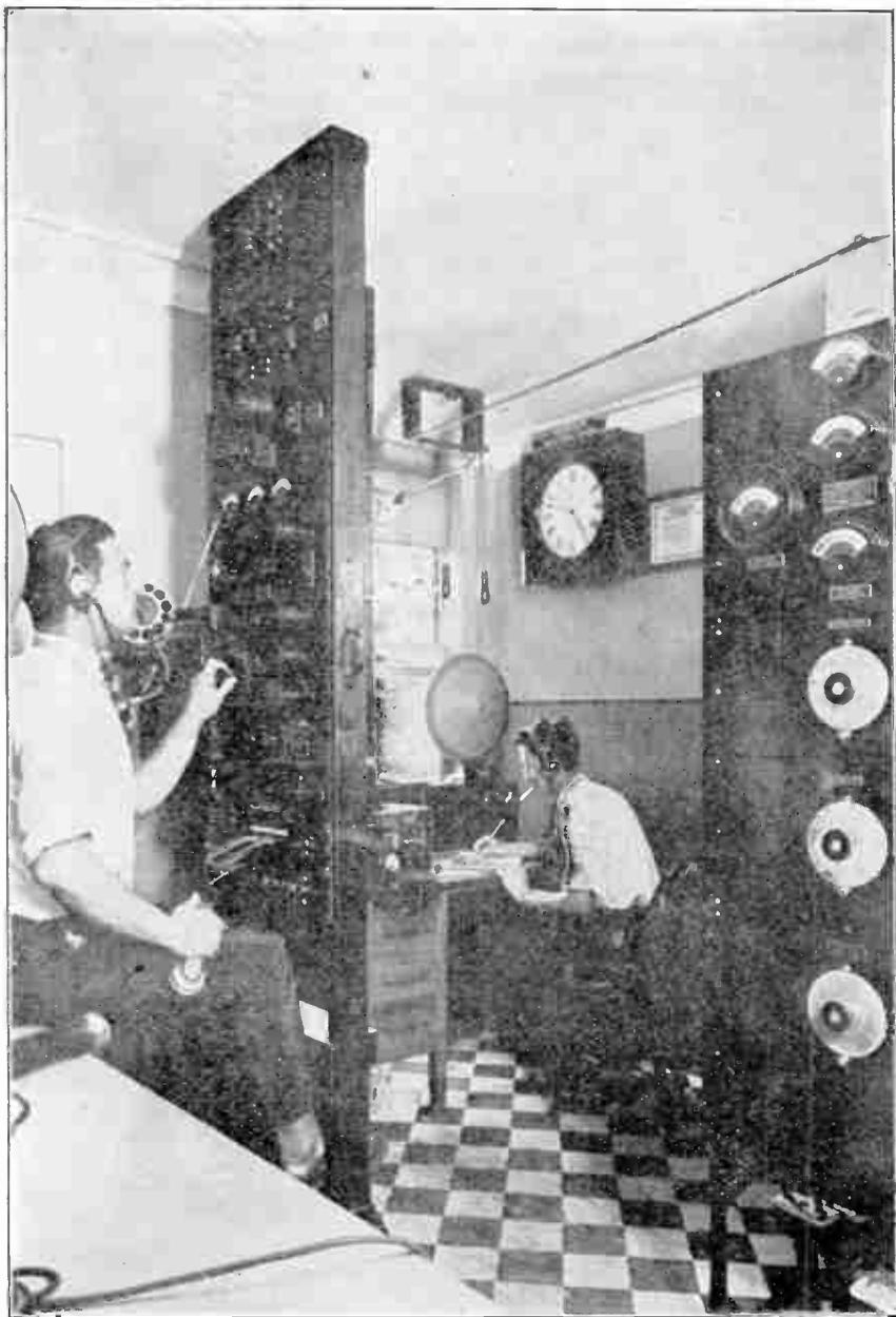
Typical control room of a modern broadcast station. To the right is shown the 600 meter operator watching marine traffic in order that the station may close down in the event of an "SOS" call.
