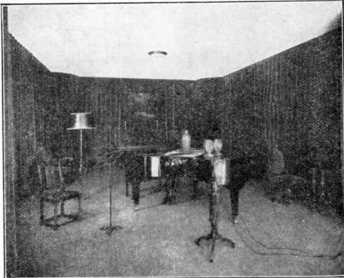
The concert studio of a radio broadcast station. Fixtures, draperies and furnishings are so arranged to give the best acoustic properties. Note the two microphone transmitters on the pedestal.
