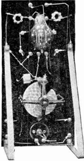
Rear view of a short wave amateur transmitter showing methods of construction, keeping the leads short and straight in the vital parts.
