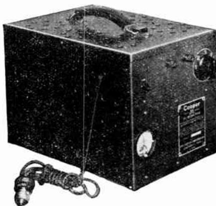
A rectifying tube type of "A" eliminator, the output voltage of which is adjustable.
