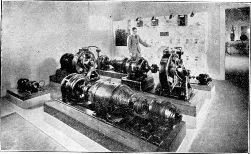
Generator room of an up-to-date radio broadcast station. Note the spare set of generators.
