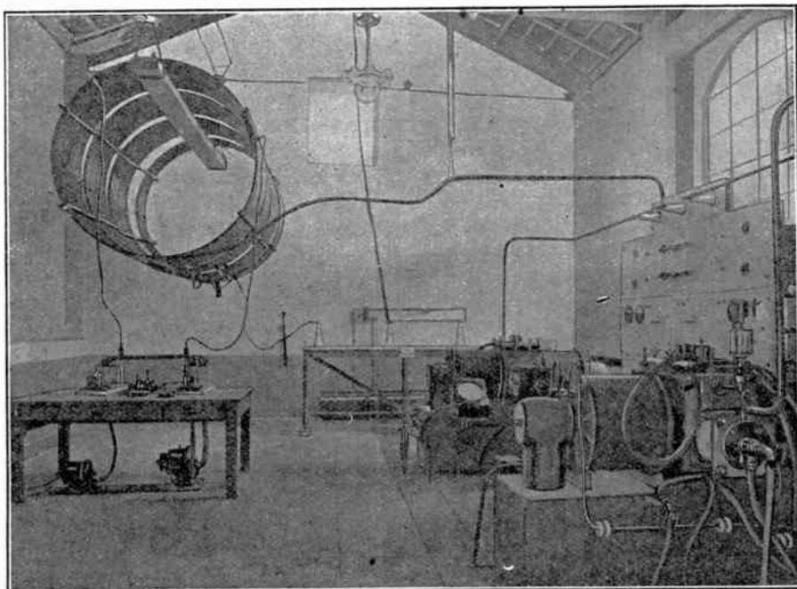
The high power station at Rome, Italy. Two powerful arcs are used to supply the energy to the aerial.
