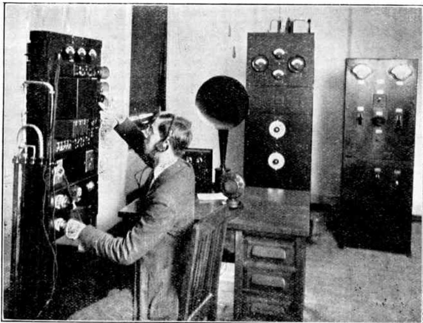
The operator "listens in" on a monitor and governs the modulation by means of a potentiometer. The tall machine in the rear of the room is the radio transmitter, to the right is the power panel.
