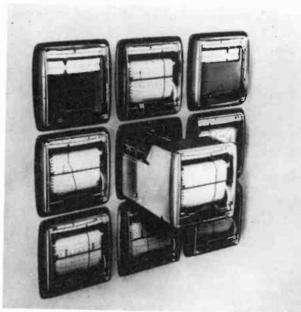
*Fig. 1019. This bank of recorders is installed on slides easily accessible for maintenance.*
