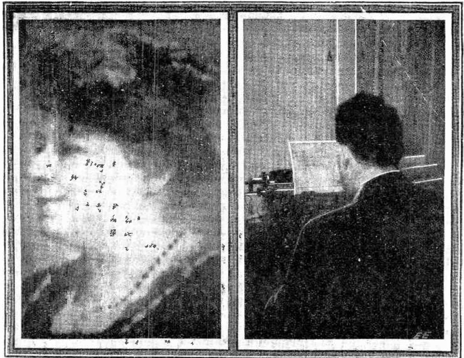
Fig. 15. At the left a reconstructed picture is shown, which was telegraphed by code letters over a long telegraph line. The right-hand photo shows Dr. Korn reconstructing this very picture from a code telegram on his special typewriter, each key of which has a dot of certain size on it. Instead of a letter, these varying dots make up the picture.
