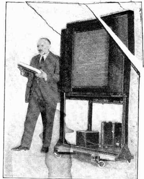
Fig. 96. Dr. Herbert E. Ives is shown holding one of the giant photo-electric tubes. At his left, the screen on which the large television image was reproduced.
