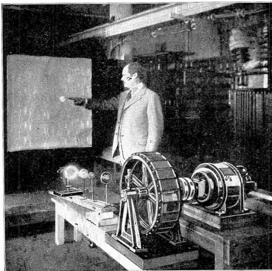
Fig. 78. Dr. Alexanderson in his laboratory indicating the seven light-spots, which are used in the method proposed by him for television. In the foreground is the drum on which are mounted the mirrors, with the motor for rotating it. A system of lenses may be seen, together with an arc light.
