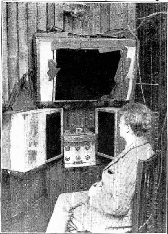
Fig. 88. Mr. Baird seated before his television transmitter. The three black-faced boxes are the sources of the infra-red rays.
