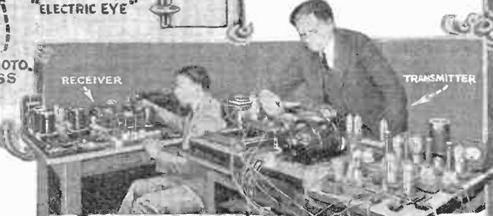
The receiving station where the apparatus is in absolute synchronism, records the photos in three ways, by tape, by pen sketch and photographically. Above: Complete outfit.
