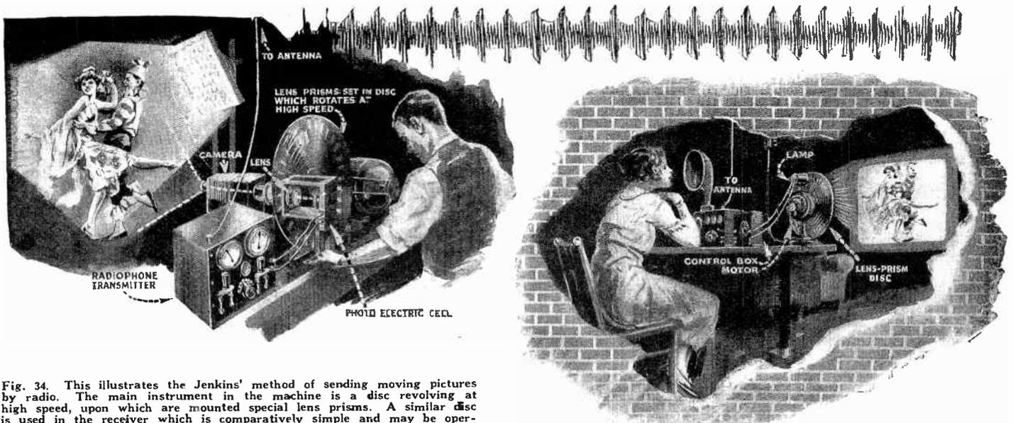
Fig. 34. This illustrates the Jenkins' method of sending moving pictures by radio. The main instrument in the machine is a disc revolving at high speed, upon which are mounted special lens prisms. A similar disc is used in the receiver which is comparatively simple and may be operated from an ordinary radio receiver and amplifier.
