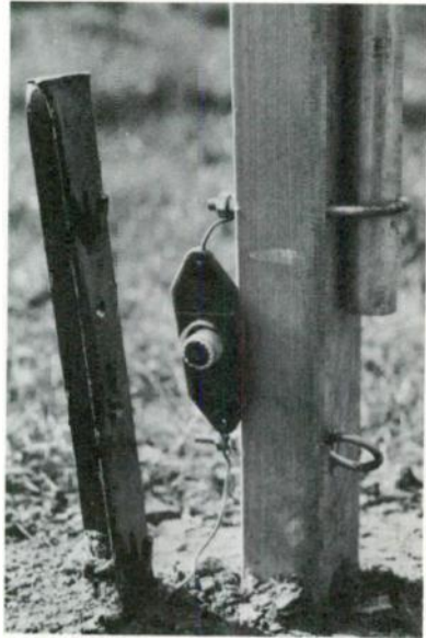
Fig. 51. Base construction for each of the four-square verticals.
