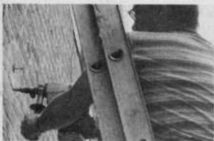
Fig. 7. While a saber saw can be used to cut through a frame outer wall, something a lot heavier is needed for brick. You can hack away at the brick with a cold chisel and sledge, but a few dollars spent to rent an electric hammer (with chisel bit) will let you bust out the wall in minutes. Note the screw sticking through the pilot hole, used to center the duct circle scribed with chalk.
