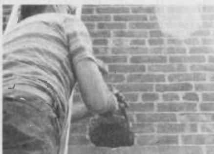
Fig. 8. The final trim is done by hand with a cold chisel and small sledge. The sheet metal duct should just slide through the hole without bends or a force fit. Chip away small bits of brick until the duct can slide in and out easily.
