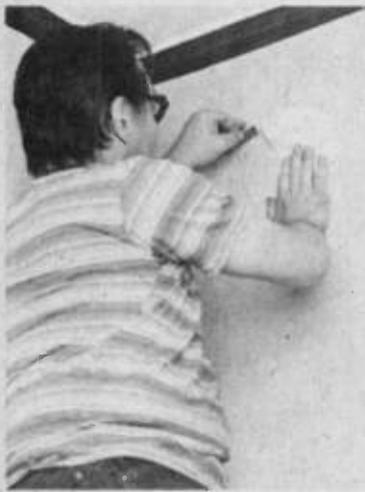
Fig. 1. Pick a location for the grille-damper, and make certain it's between two wall studs. Using the duct as a template, scribe the outline on the wall and then use a razor to cut away the wallpaper.
