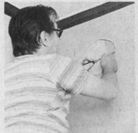
Fig. 3. If the wall is plaster, scribe the outline and then chip out the plaster until the lath is exposed. The lath can be either strips of wood, wire mesh, or plasterboard—a sheetrock-type material with a pattern of large holes into which the plaster locks when dry.
