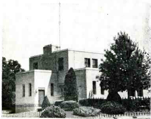
This Mosley V-27-GP antenna is perched atop the administration building of the Calvary Cemetery in St. Louis, Mo. Mobile units maintain continual contact with the superintendent's office, using Citizens Band radio throughout the cemetery's 425 acres.
