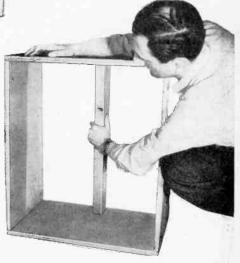
2 Rear 2" x 4" brace is placed with narrow side flush with rear edge of top and bottom panels. Two #8 flat-head wood screws and glue should be used at each end to hold 2" x 4" brace in position.
