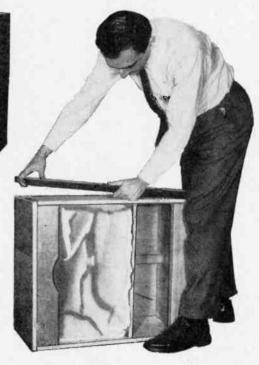
**5** Finishing panel, although not necessary, may be added for the sake of appearance. Four wood screws through cabinet hold 30" x 16" panel in place. Interior of top compartment should be loosely lined with Fiberglas, rock wool, or other acoustical damping material. Cabinet may be used upright as lowboy, finished or unfinished, as desired.
