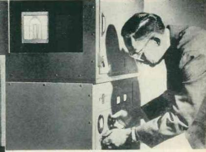
Electronic light amplifier, left, increases projected light's brightness 1000 times. Potential lies in electronic display, radar, etc. The amplifying fluoroscope, photograph above, can increase brightness of X-ray image up to 100 times.
