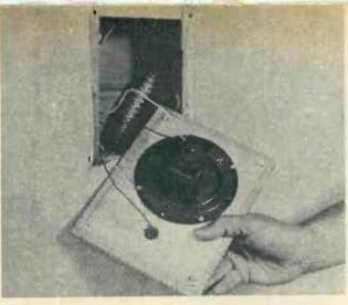
Now attach speaker and buzzer wires. Ideally, you'd have stations wired in when your house is under construction.
