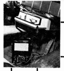
The job is done. The recorder is about 3 in. deeper than the chassis; therefore, operating push buttons, level meter, volume control and speaker will protrude just the right distance. Cement a small magnet on back of mike so it can be held to dash when not in use. To remove recorder for use in home, loosen underchassis screw, disconnect power plug and slide unit out.
