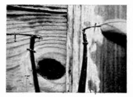
Fig. 6—Spread slit (so it matches rhombic's impedance) of twinlead 3 in. and attach to rhombic's legs. Shown here is our installation in attic.
