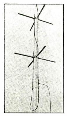
Fig. 7—Individual layers are connected together by means of two concentric lines which spiral around the pole. A simple matching network is also shown.
