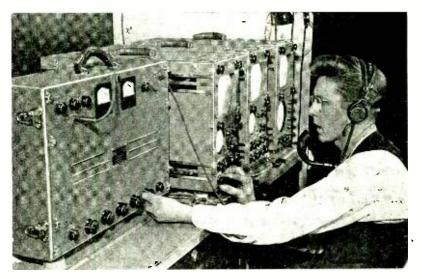
Fig. 7-Television Control Set-up at Madison Square Garden, 1944. (Audio Amplifier on Left, Transportable Orthicon Control Units on Right.)
