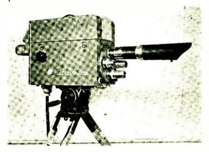
Fig. 9-The image orthicon camera.
