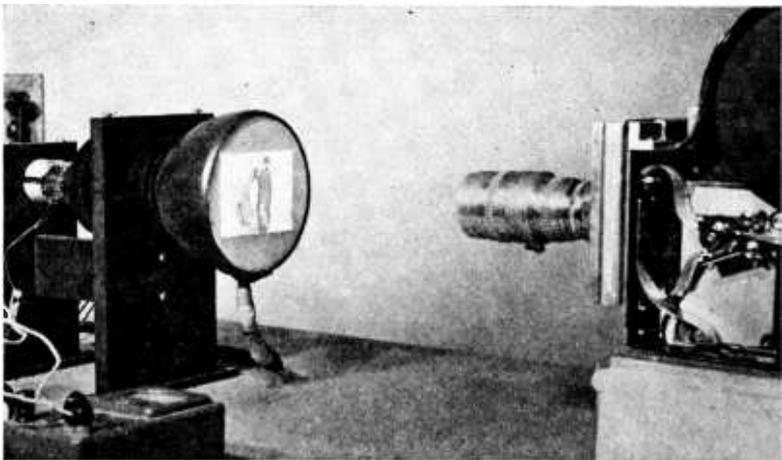
Fig. 6—Close-up of the kinescope with cover removed. (On the tube face is an actual television image of a baseball pickup.)
