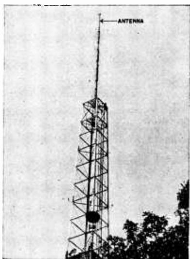
Fig. 2—The high-band antenna mounted above the WNBW Superturnstile.
