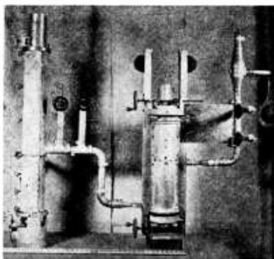
Fig. 5—500-900 Mc driver and rf power amplifier.
