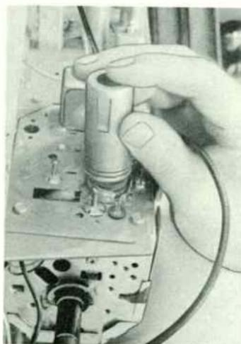
**Coupling stray fields to mixer tube by body capacitance.**
