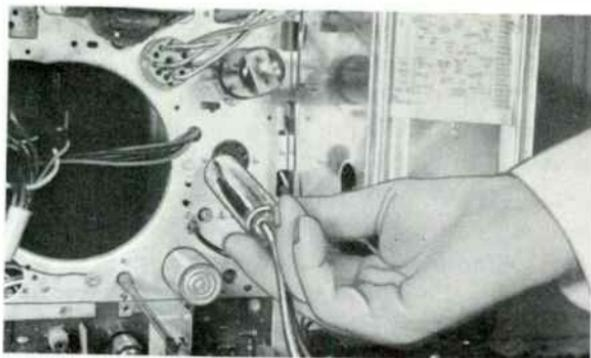
Checking drive to horizontal-output tube.
