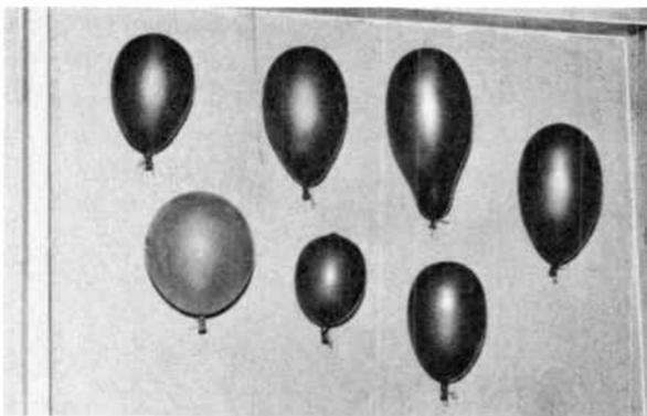
**Fig. 3-2.** A static charge imparted to the rubber balloons causes them to be attracted to a dry wall.
