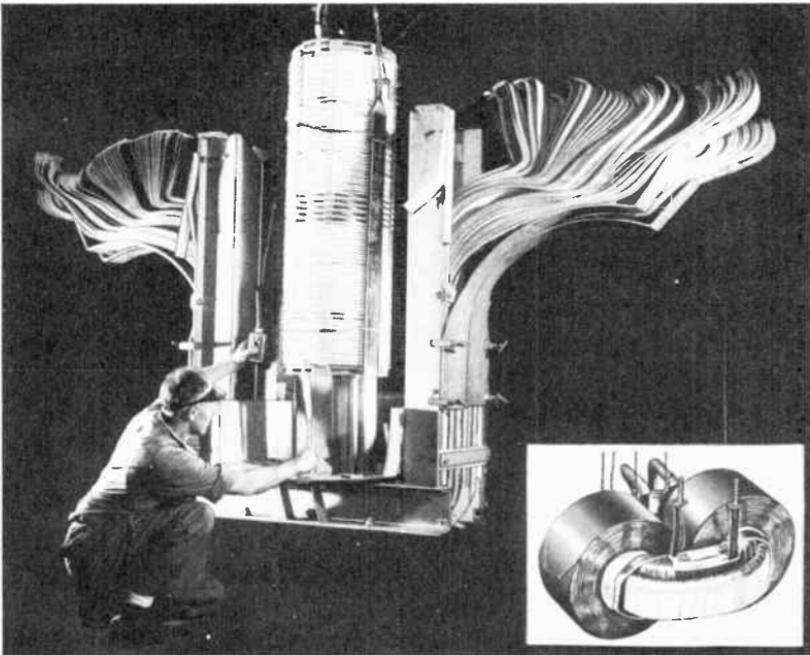
Fig. 11-13. A power transformer being assembled from a precut, preformed core of laminated steel strips. A small Spirakore transformer is shown in the insert.
