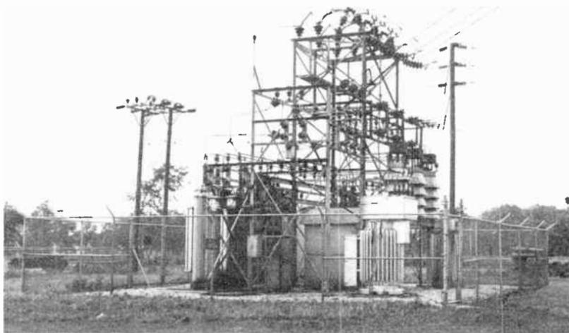
**Fig. 11-40. A typical substation where several power transformers are used. (Courtesy of Kuhlman Electric Company.)**
