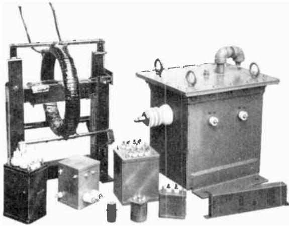
Fig. 11-14. Small high-voltage transformers. (Courtesy of Raytheon Mfg. Co.)
