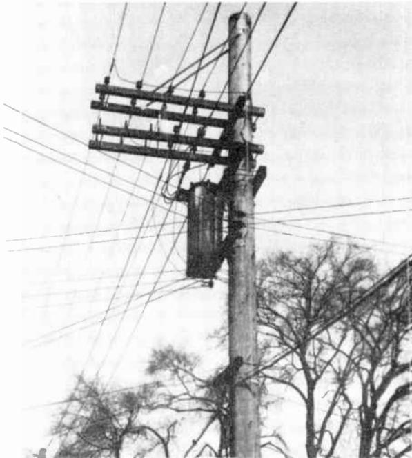
**Fig. 11-39. A distribution transformer mounted on a pole.**
