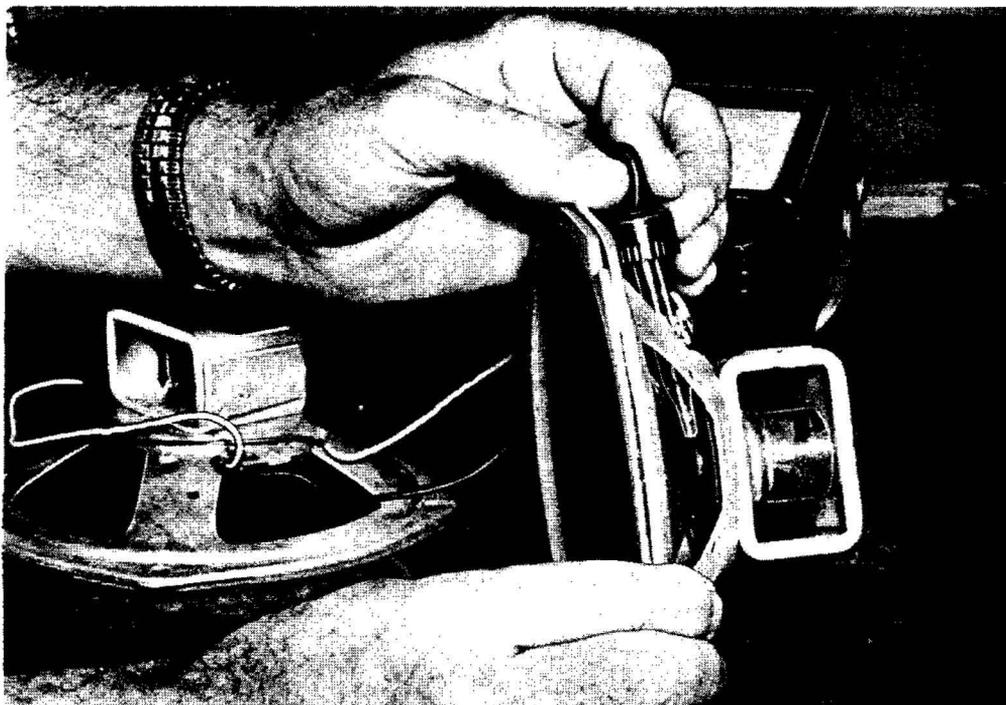
**Fig. 10-2. Applying acetone to loosen spider of a speaker.**
