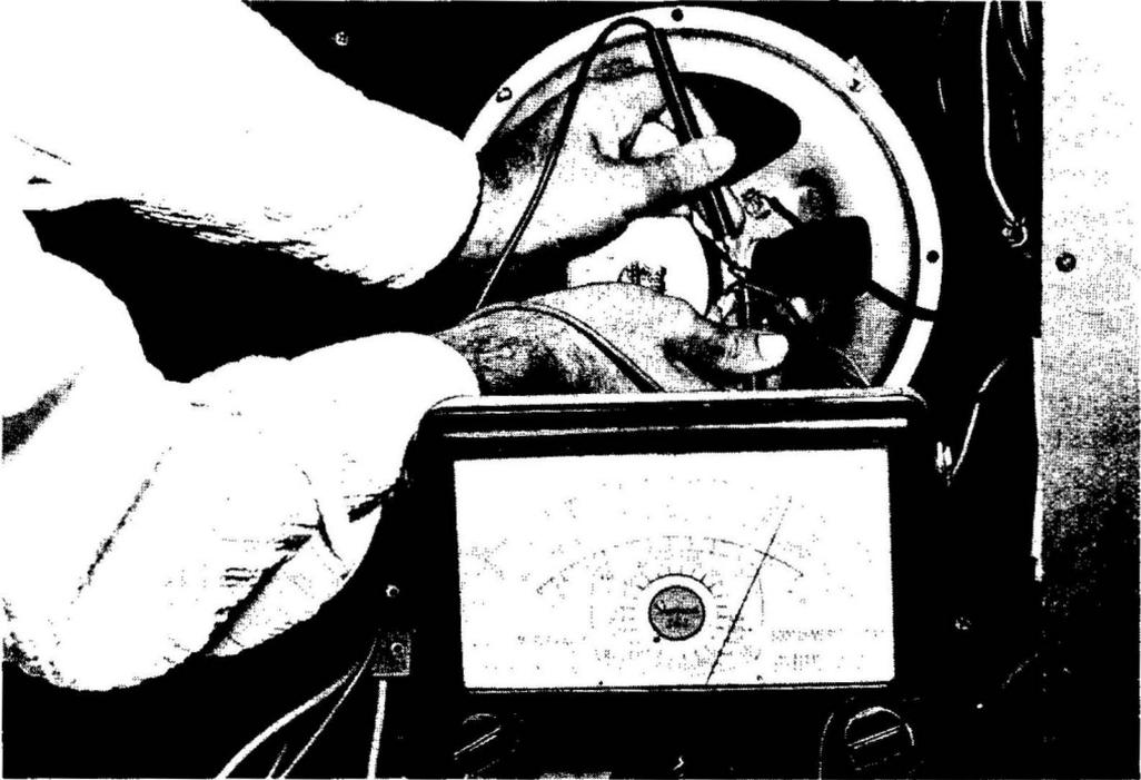
**Fig. 11-4. Testing continuity of speaker field.**
