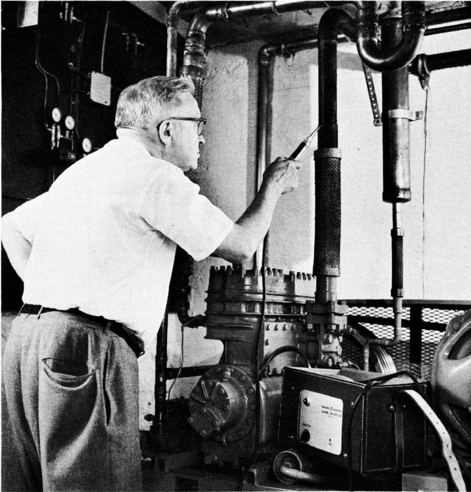
Fig. 7-65. Gas-leak detector in use. (Courtesy of General Electric Co.)
