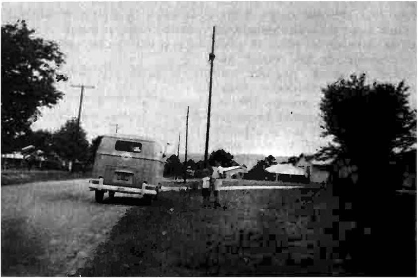
**Fig. 4-14. Searching the area with service truck for noise source, using probe dipole and field-strength meter.**
