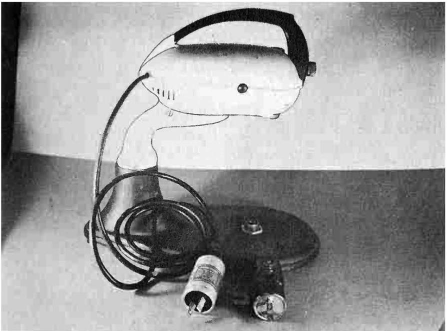
Fig. 6-5. A kitchen mixer and two plug-in line filters.
