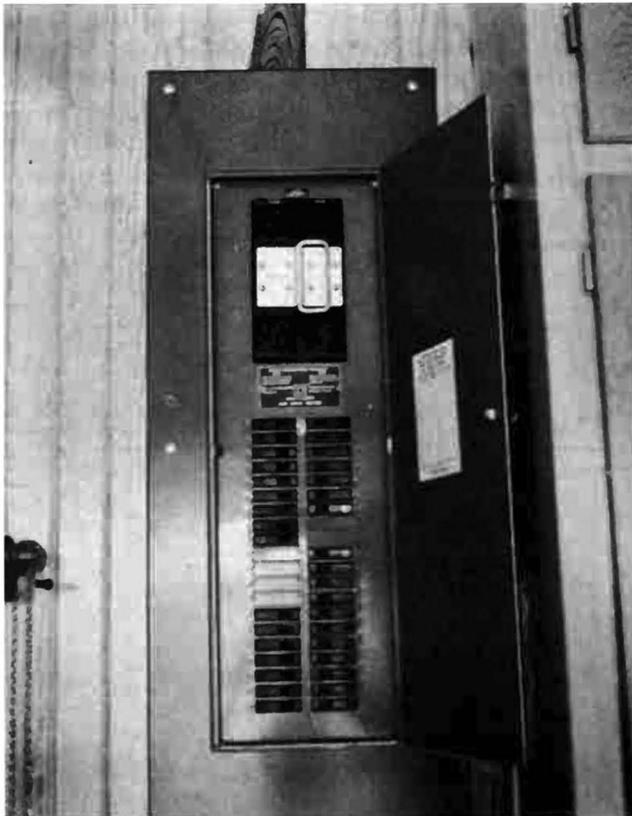
Fig. 4-5. The "breaker box" in a large house.
