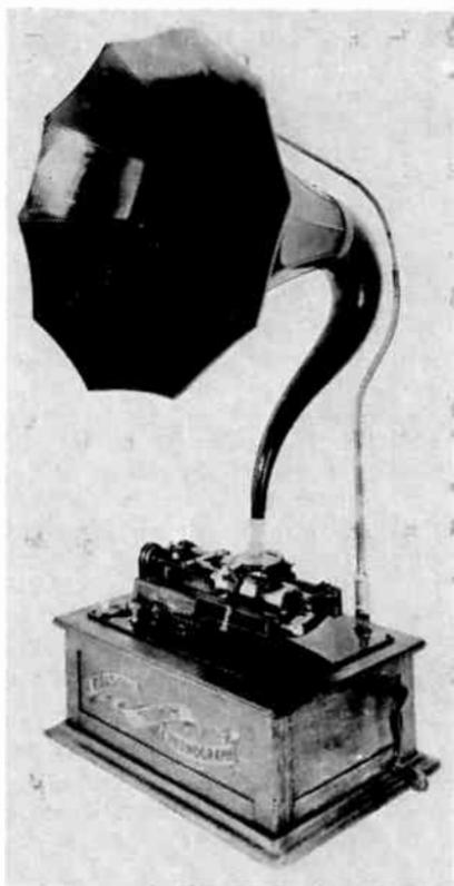
Fig. 14-3. Edison Triumph phonograph with Cygnet horn. It had a triple spring motor and speed regulator.
