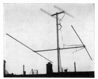
FIG. 21-2. High-low band antenna. Short folded dipole at top of mast is for channels 7 to 13; long straight dipole below is for channels 2 to 6. (From McGraw-Hill motion-picture series, Basic Television.)
