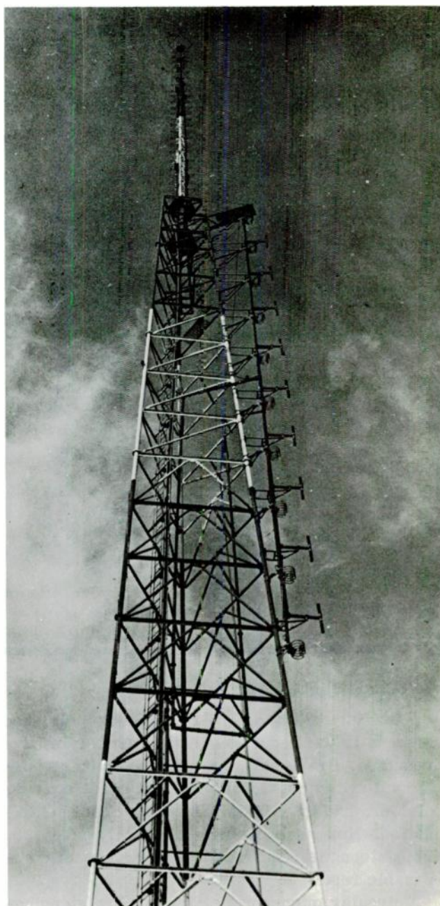
Fig. 8-5. Dual polarized antenna radiators side-mounted on an existing TV tower as an interlaced system.
